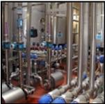
When the beer is sufficiently mature, it is filtered to remove remaining solid particles from the beer. Distinctive parameters are the circuit, the beer, CO<sub>2</sub> and sugar levels. Every 2 seconds, 15 analog values are monitored.
